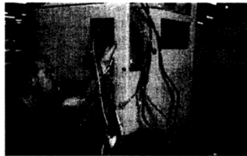
Fig. 5 Cable harnesses within an electro-mechanical assembly.
